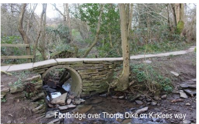
Footbridge over Thorpe Dike on Kirklees way
